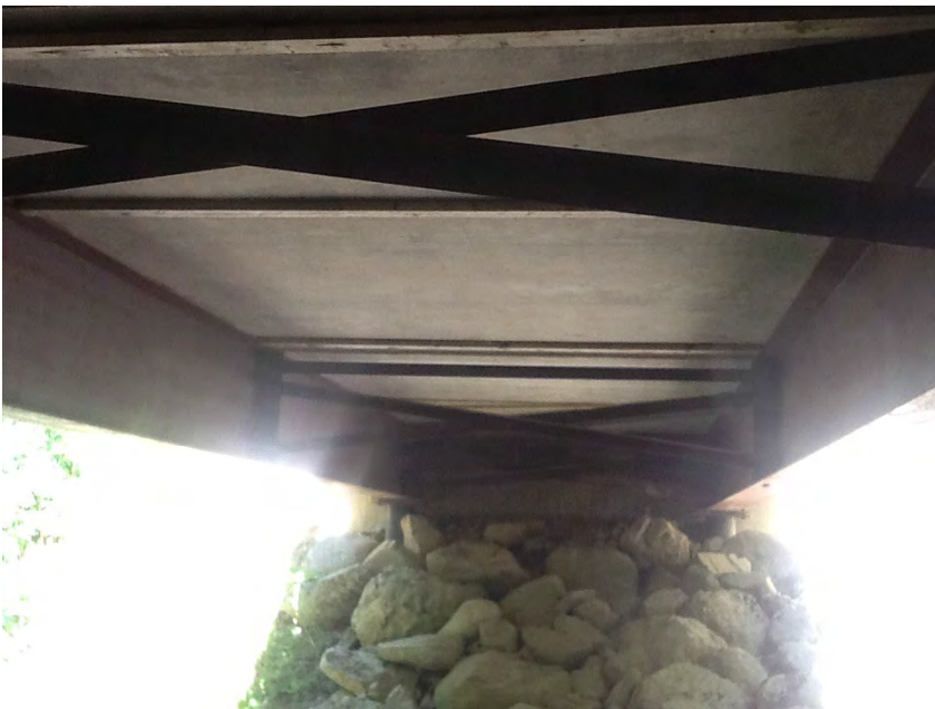
Underside of bridge
