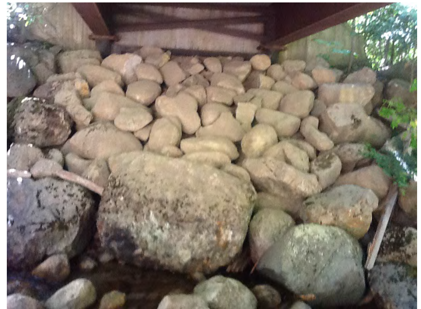
Left Bank Abutment when facing downstream
