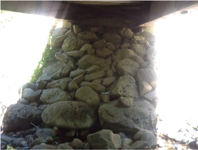
Right Bank Abutment when facing downstream
