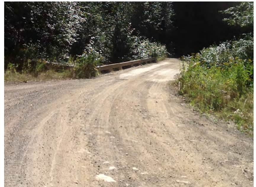
Right approach facing structure
